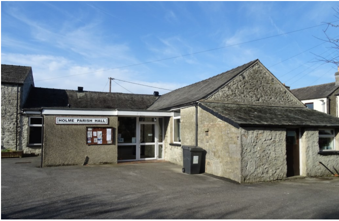
Holme Parish Hall
