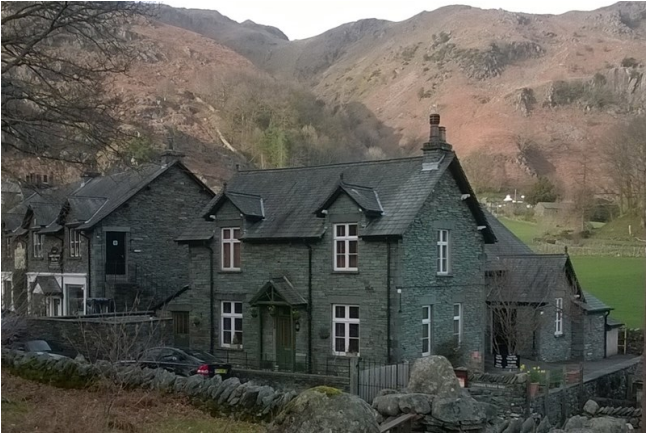
Church Hall Cottage, Chapel Stile.
