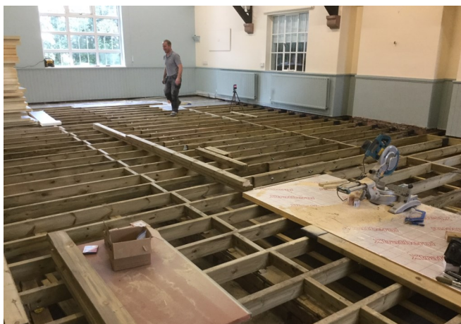
Work to replace the wooden flooring
