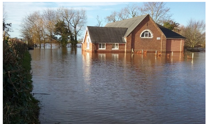
Crosby-on-Eden Parish Hall in flood water
