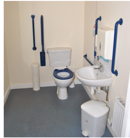
New disabled toilet facilities
