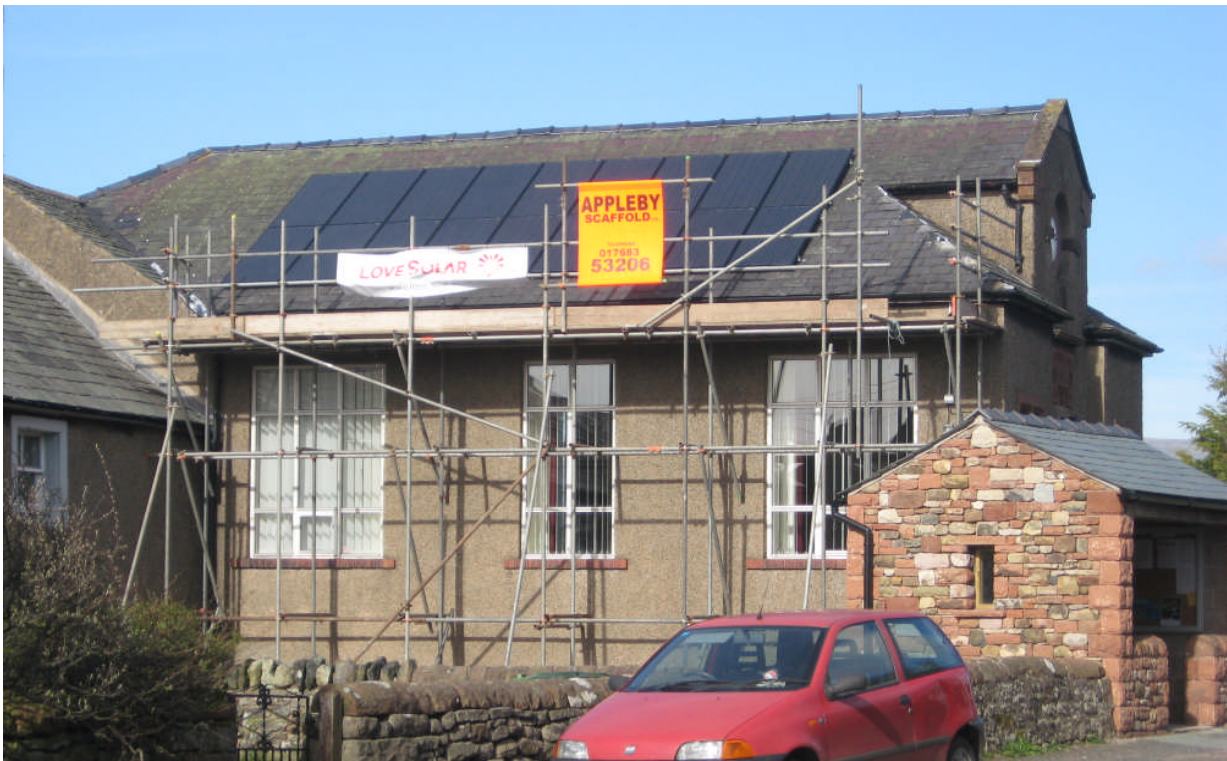
Installation of Photo Voltaic Panels on Bolton Memorial Hall
