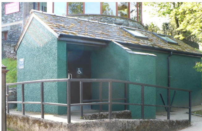
Rothay Park Public Toilets
