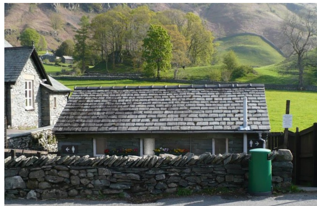
Chapel Stile Public Toilets
