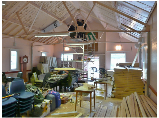
Insulation panels fitted inside the roof
