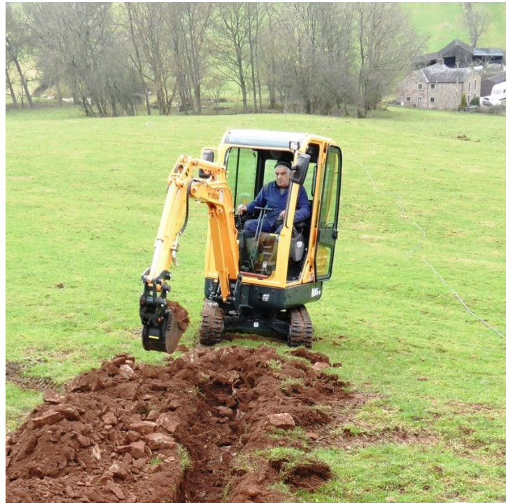
Laying cable during the network upgrade
