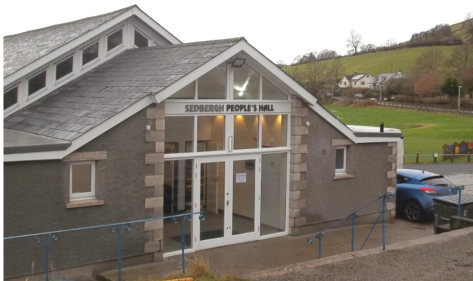
Refurbished entrance to Sedbergh People's Hall
