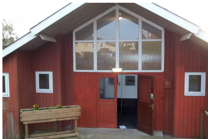
Hall entrance prior to refurbishment
