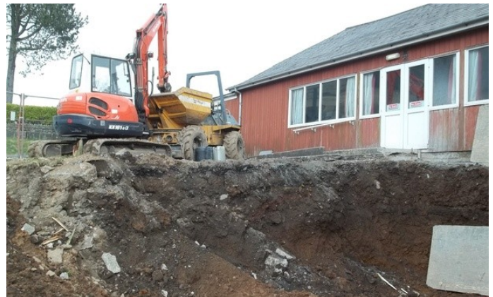
Excavating for Stage One Extension
